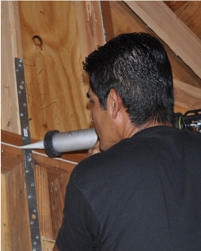
Manual Air Sealing
