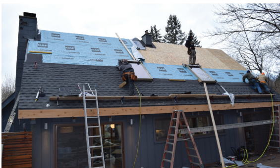
SIPs installation on the Michigan house.
