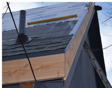
Installing the eaves troughs on the Michigan house.
