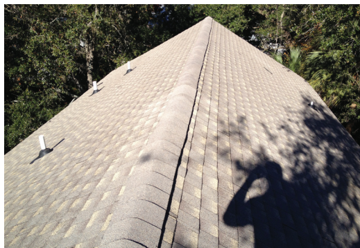
The roof once complete in Georgia.
