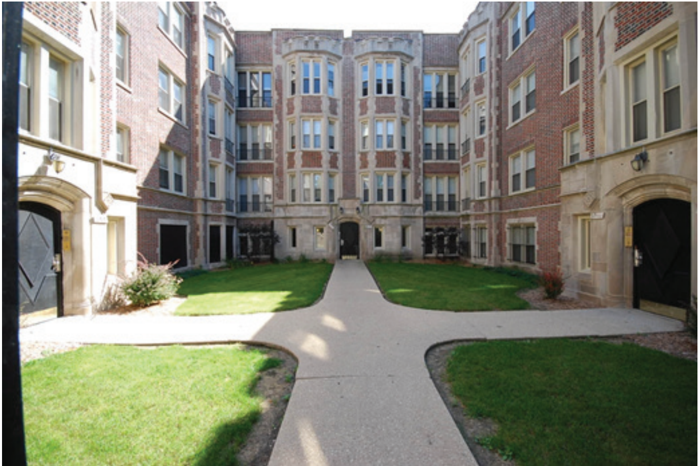
2909-29 E. 78th Street apartment building courtyard and entrance (Chicago)
